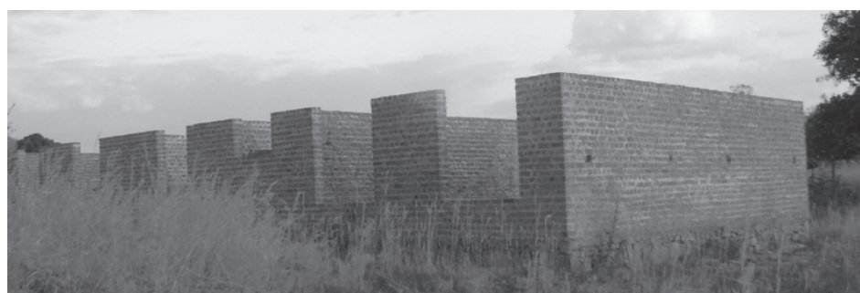
Construction on the Bethlehem Tailors Training Centre
